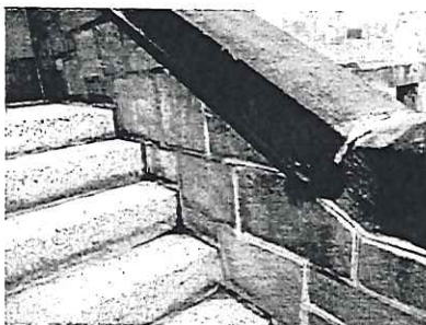
Missing mortar at stairs
