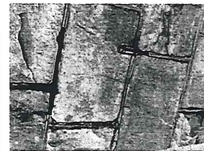
Missing mortar in stonework
