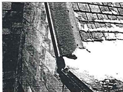
Evidence of slate roof tiles slipping.
