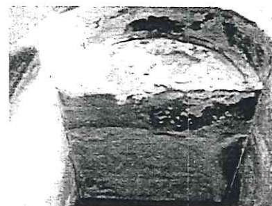
Close-up view of delaminated / flaking brownstone above south facing entrance door
