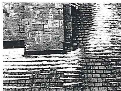
Worn slate roof tiles
