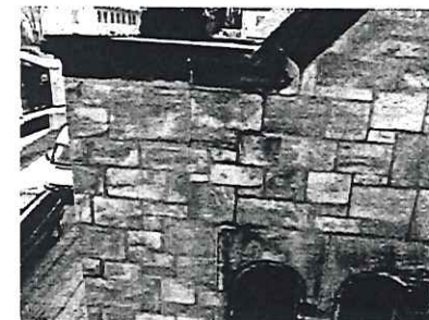
Cracked stone and cracked mortar
