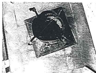
Uncovered top of flue stack
