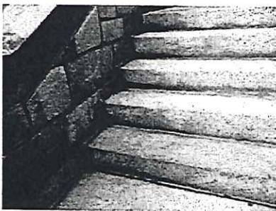
Missing mortar at stairs
