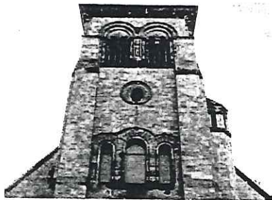
Tower east elevation. Cracked capping stone on east wall of both north and south wings.
