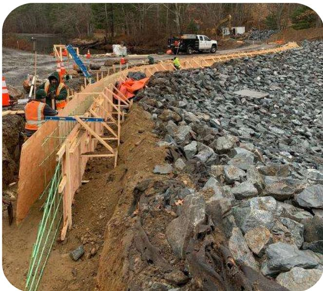
The dam repairs brought this structure into compliance with the MA Office of Dam Safety Standards through repairs to the flume box structure, headwalls, construction of upstream and downstream cutoff walls and the armoring of the upgradient and downgradient slopes.
