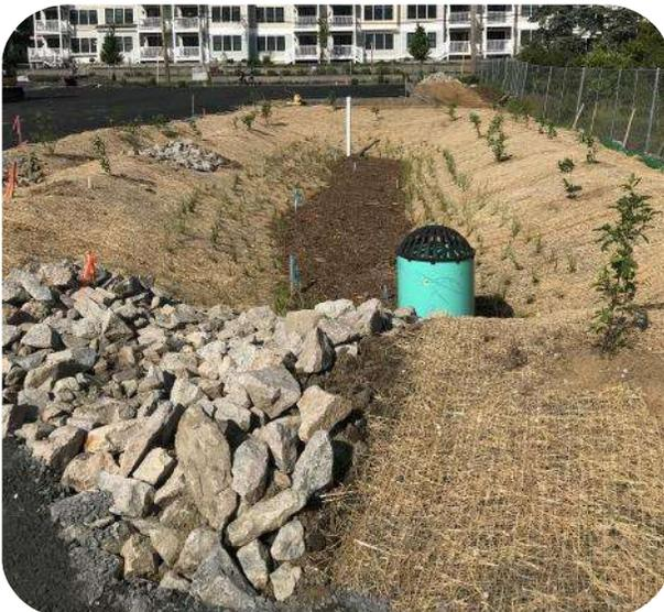
This project involved the capping of zinc-contaminated soil underneath a parking lot between Plymouth Harbor and Water St. Ongoing storm damage to the site was creating the potential eco-hazard risk of this material entering the harbor and bay. By capping the site, rebuilding the coastal revetment and removing the traditional stormwater system in favor of a bioretention facility DMEA was able to stabilize the site and protect our marine environment.
