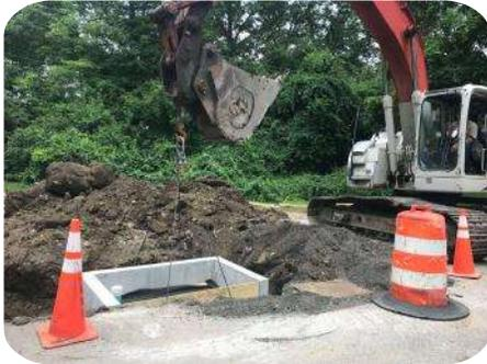
This project was identified in a study as having one of the larger stormwater inputs into Great Herring Pond. DMEA received grant funding for design and construction to install dozens underground recharge areas within the roadway to infiltrate and treat the stormwater prior to reaching Great Herring Pond. The project also includes a raingarden for further treatment prior to discharging. The project has been widely successful.
