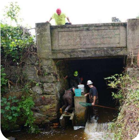
The project was done in conjunction with the upstream Holmes Dam removal and stream restoration. The new bridge is a box culvert allowing for fish passage and resiliency to climate events. Along with a new bridge, stormwater, sewer and water utilities were upgraded along with sidewalks, landscaping and a restored stream channel improving aquatic habitat and fish passage.
