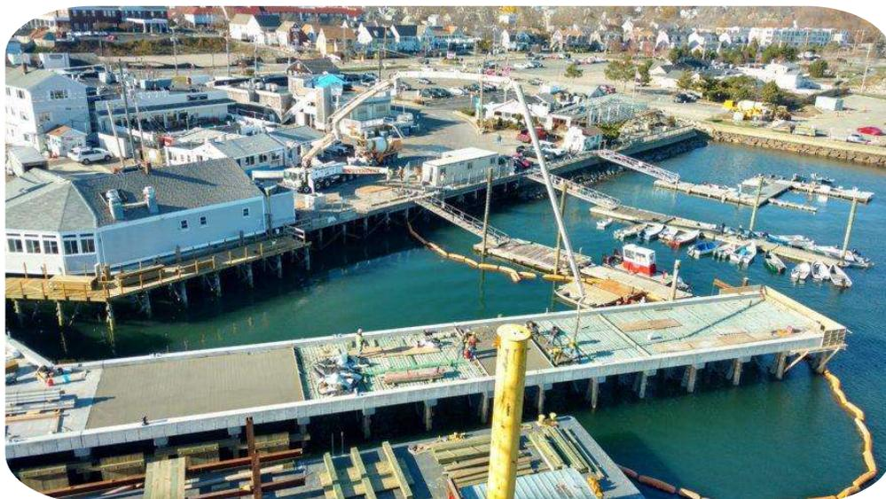
DMEA partnered with the Commonwealth to reconstruct the T-Wharf and make it available to the commercial fleet as it had been closed for several years due to its poor condition. It is a completely new structure with stormwater controls, winches, lighting, berth space and plenty of open area for use.
