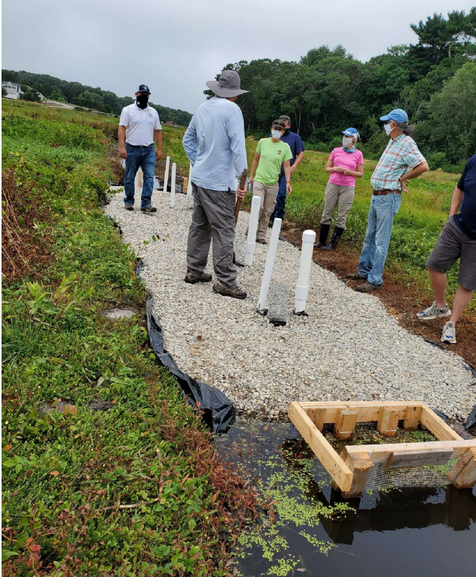
Figure VI-2. Experimental In-stream PRB. Permeable Reactive Barrier (PRB) installed in a cranberry bog stream in Barnstable, MA. Installations of these types of PRBs require performance monitoring, consideration of design characteristics to ensure flow-through and avoid upstream flooding, and selection of PRB media to remove phosphorus. Photo courtesy of A. Unruh, Town of Barnstable.
