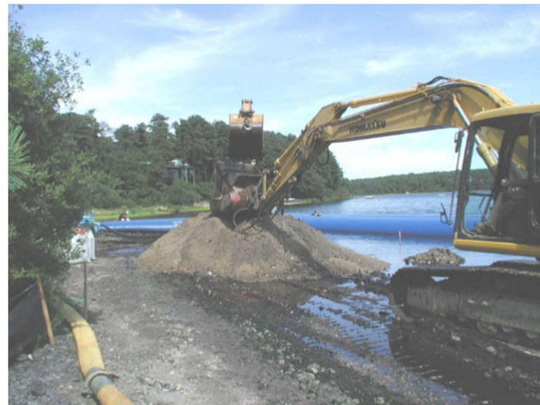
Figure VI-4. Ashumet Pond Phosphorus Plume and Excavation and Dewatering to install Iron Filings PRB to treat phosphorus. P concentrations in plume were > 5 mg/L. PRB was installed along ~300 ft of shoreline. From CH2M Hill (2005).
