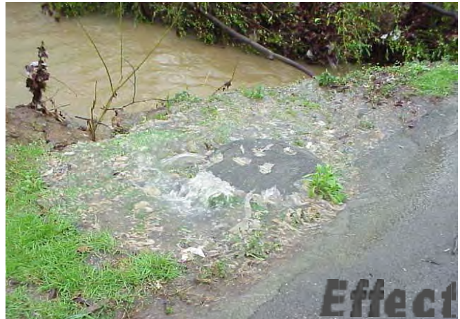
Sanitary Sewer Overflow Caused by Grease Accumulation
