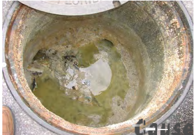
Grease Accumulating in Sewer Manhole
