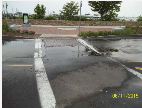
Groundwater seeping up through pavement
