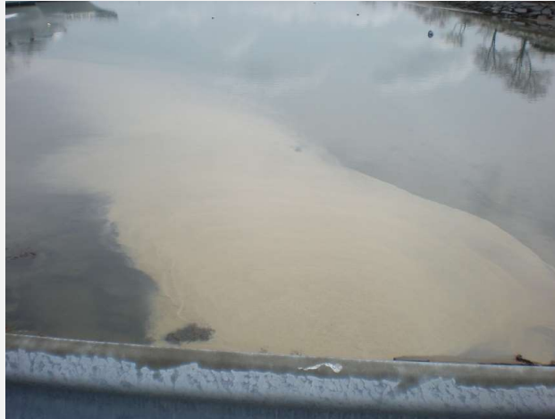
2014 Installation: Pumped Water and Sediment from Construction Activities into Harbor
