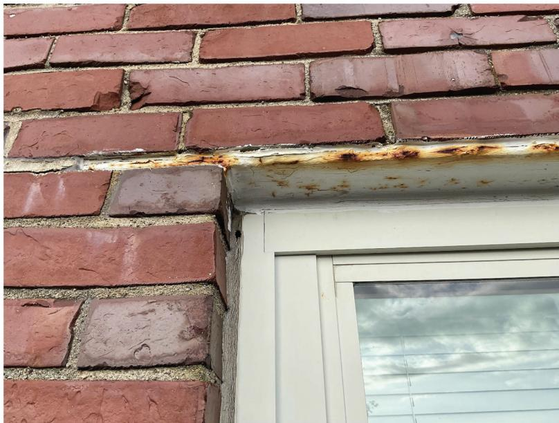
**Example of damage due to no weep holes or other arrangement for water to drain. Typical around building**
