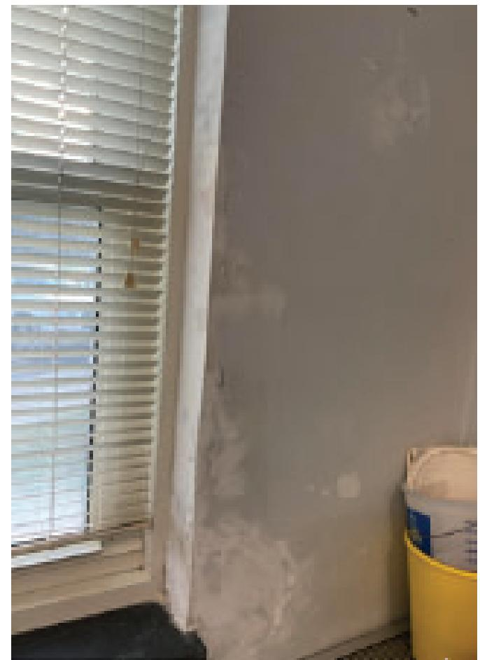
**Samples of internal building damage due to water taking the path of least resistance to inside the walls.**
