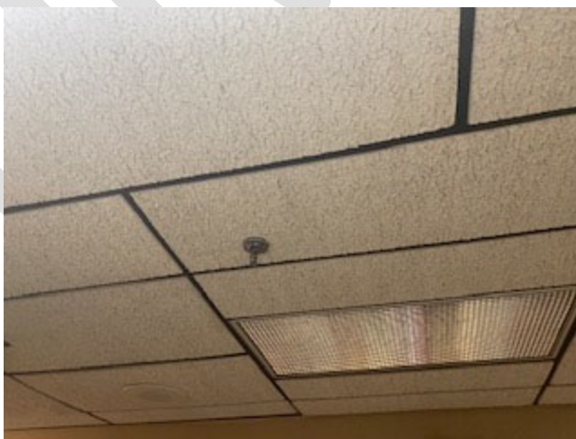
Sprinkler and Ceiling Tiles (Typical)
