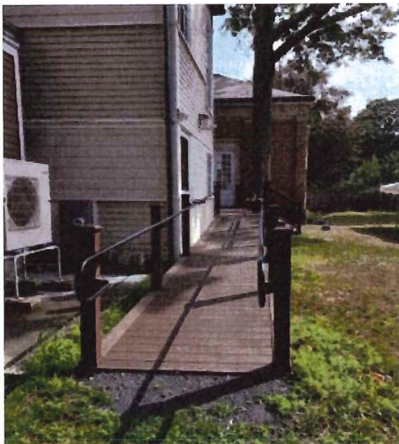
Rear Accessibility Ramp – Needs Cement Pad Landing
