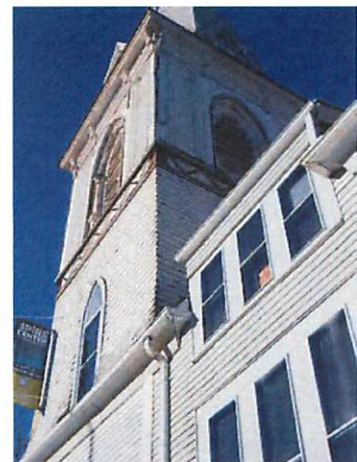
Aluminum gutter and downspout at the east elevation.
