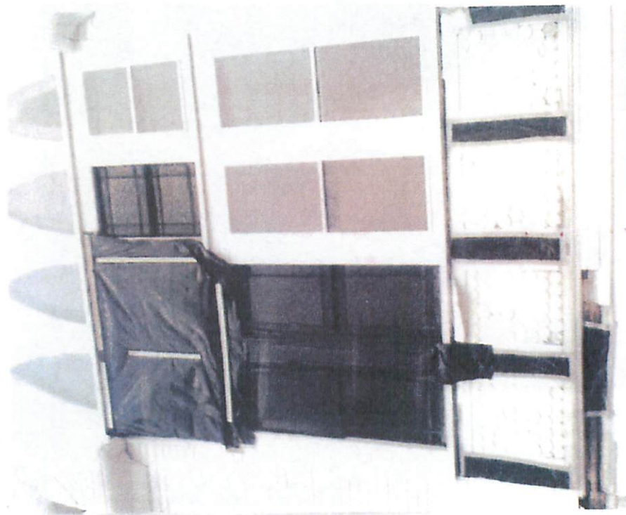
Figure 7c. Spire Center for the Performing Arts, Plymouth, MA. West transept gable - exploratory investigation of structural conditions. Photo: Lynne Spencer
