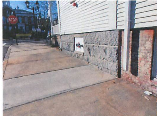
Dressed granite-faced brick foundation at southeast tower.
