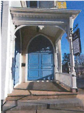
Left: Arched double entry with molded trim. Curved and carved roof brackets and carved porch posts and balustrade. Right: Oculus window at transept gable.
