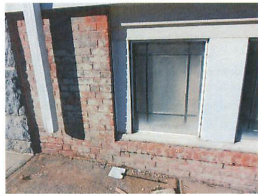
Failed mortar and paint remnants at east elevation.
