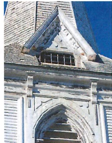
Worn and missing wood shingles at the tower and spire.
