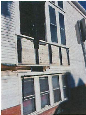
Left: Fishscale shingles revealed under vinyl siding. Right: Copper finial at southwest tower.
