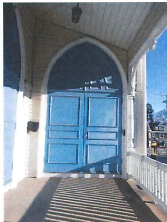
Double arched door at main entry showing weathered paint.
