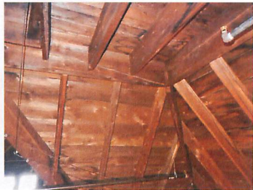
Wood framing at hip roof.
