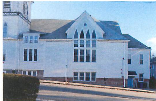
Wall surfaces and trim elements covered by aluminum siding.
