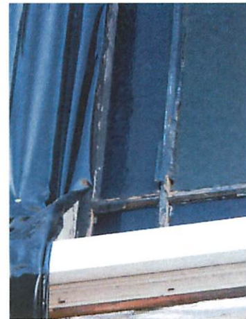
Paint failure at window muntins.
