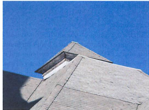
Aged asphalt roofing.
