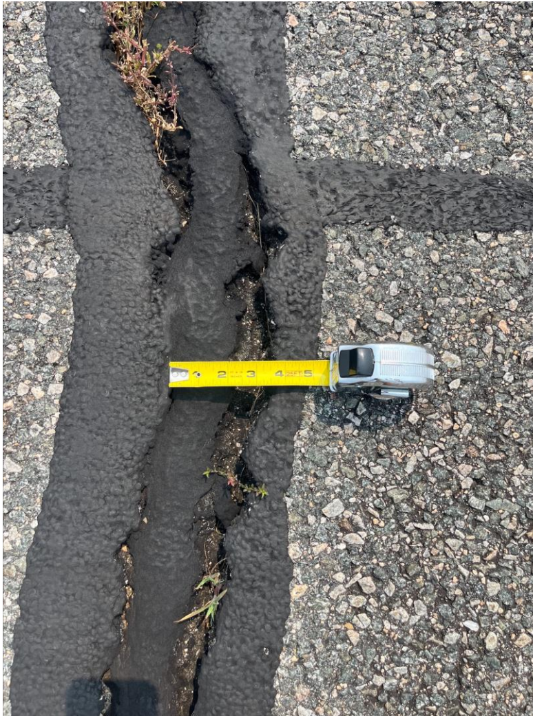
An example of a 4-inch crack that has also been crack sealed but is too large to correct the issue.
