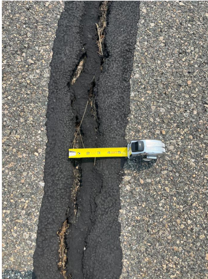
An example of one of the 3-inch cracks that has been attempted to be crack filled
