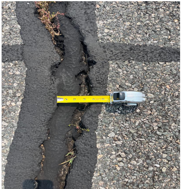
An example of a 4-inch crack that has also been crack sealed but is too large to correct the issue.
