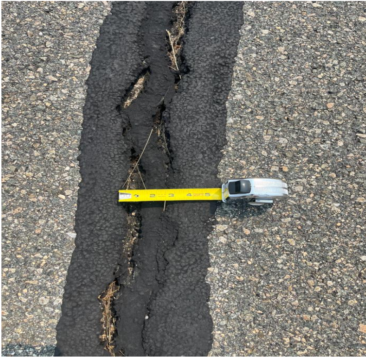
An example of one of the 3-inch cracks that has been attempted to be crack filled
